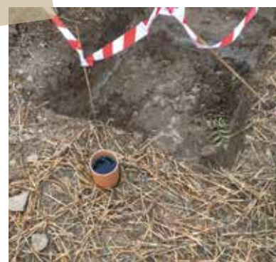
Fig 1c: Soil pipe infiltration test
